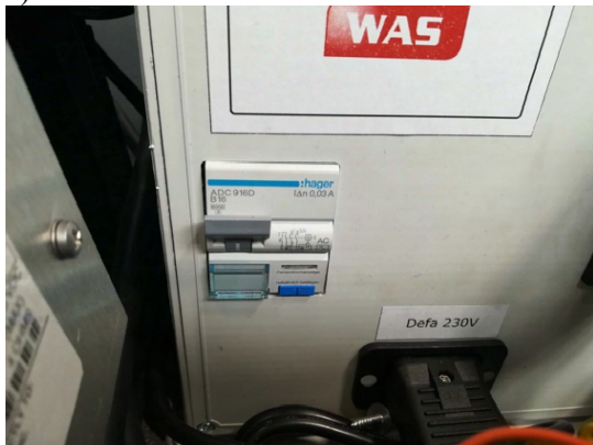
Fig. 12. a) residual current circuit breaker in the "ON" position b) residual current circuit breaker in the "OFF" position
