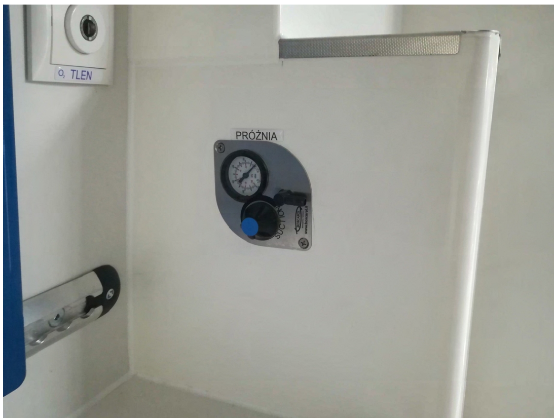
Fig. 37 Location of suction power regulator
