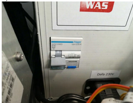
Fig. 12. a) residual current circuit breaker in the "ON" position b) residual current circuit breaker in the "OFF" position
