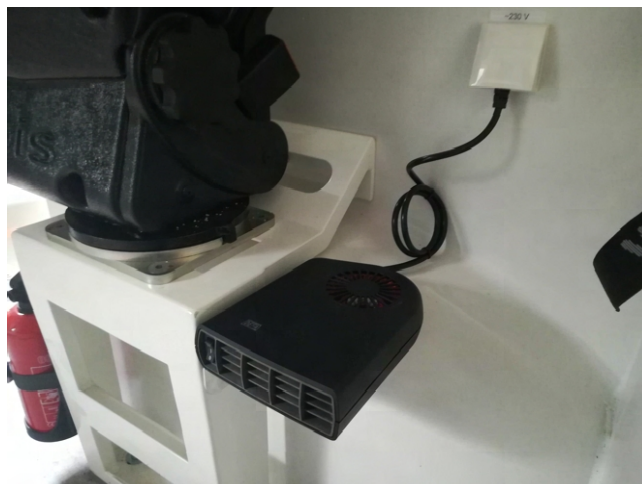
Fig. 25. Location of stationary 230V mains-powered medical compartment heater (DEFA 2100 W)
